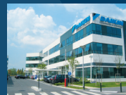
Daikin Holding USA
